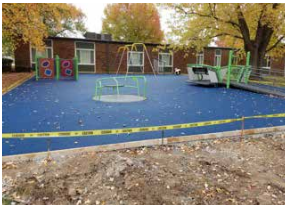
A New Playground at Camelot for Special Needs Children
